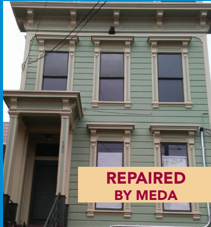
380 San Jose after repairs.
