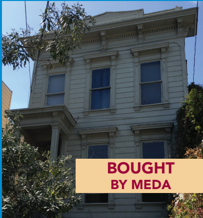
380 San Jose before repairs.
