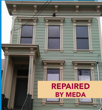
380 San Jose after repairs.
